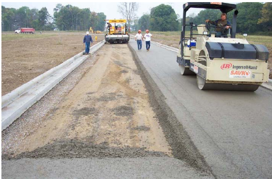
Figure 1-1 Construction of RCC pavement [1]
