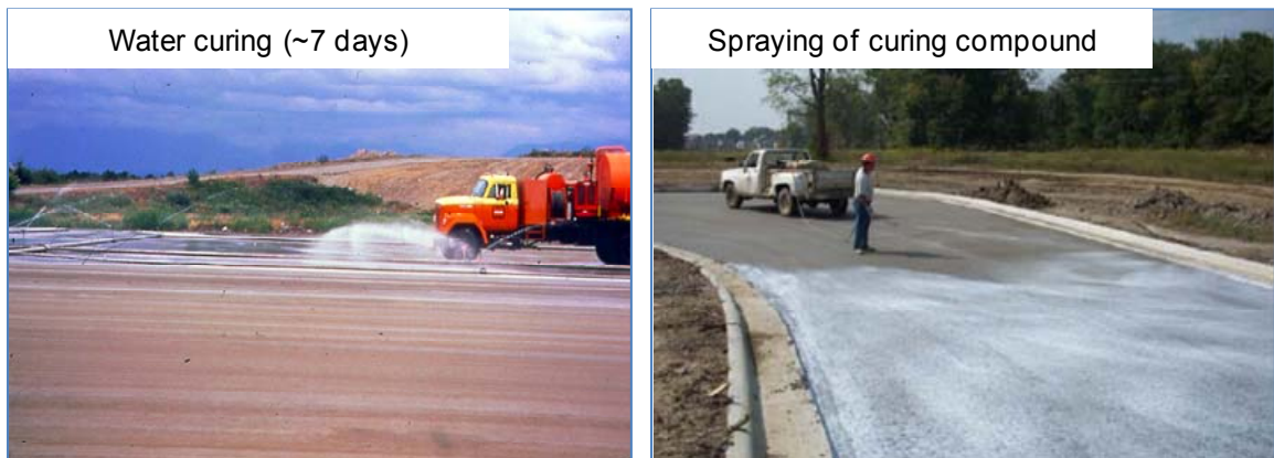
Figure B-5 Curing of RCC [30, 32]
