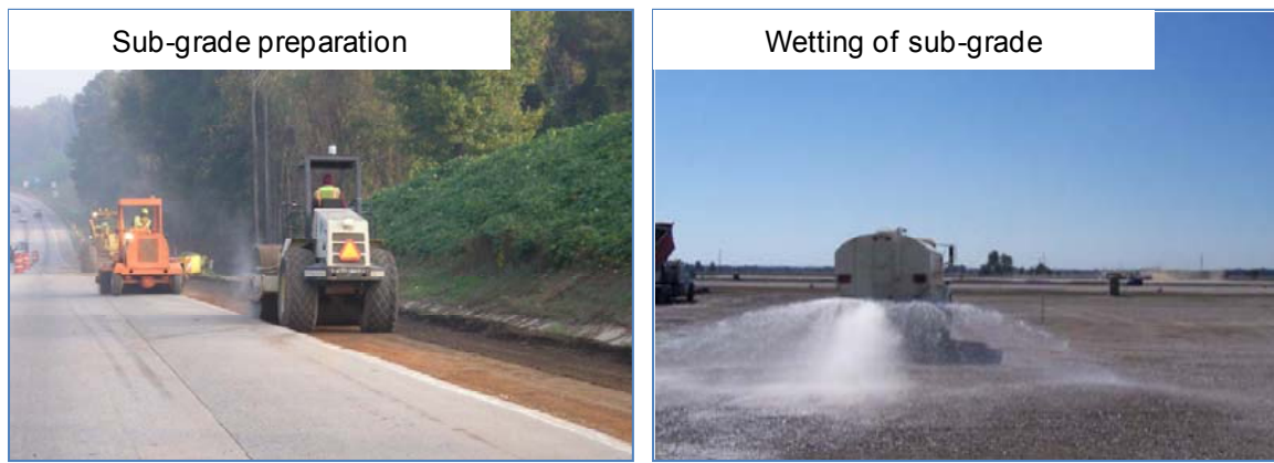
Figure B-2 Sub-grade preparation [30-31]
