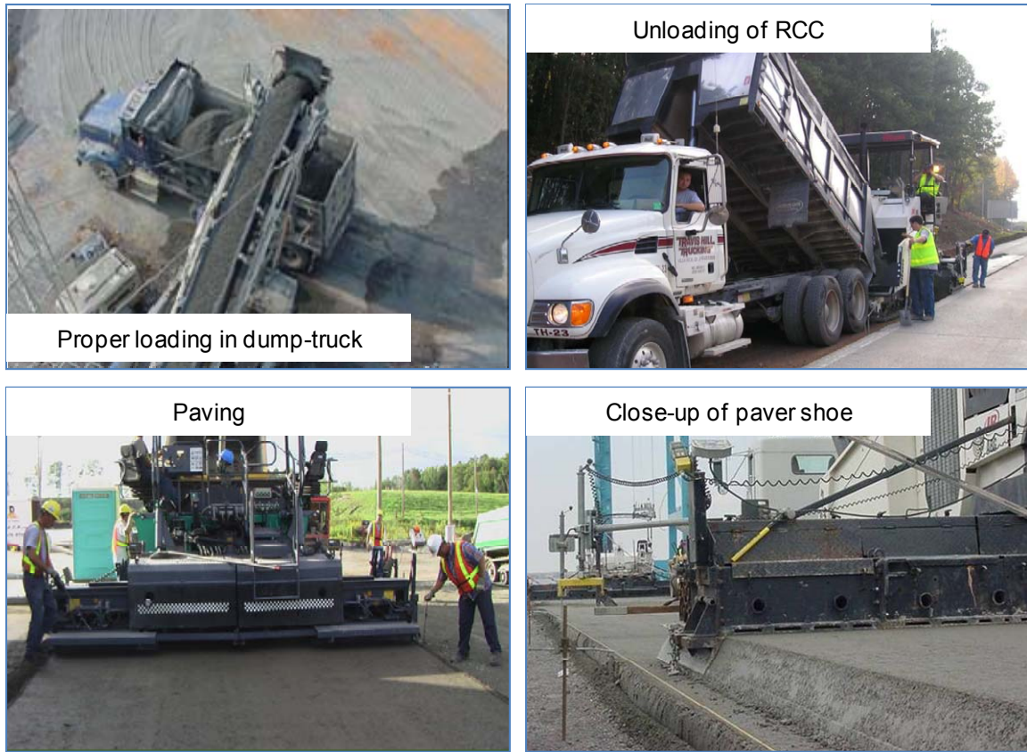
Figure B-3 RCC loading, unloading and paving [31-32]
