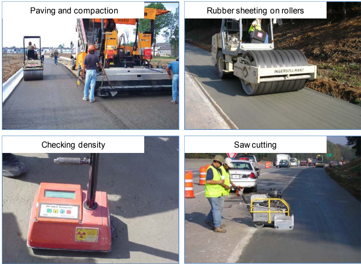
Figure B-4 Compaction, density checking, saw cutting [31-33]
